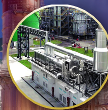
Combined Heat & Power Plants
